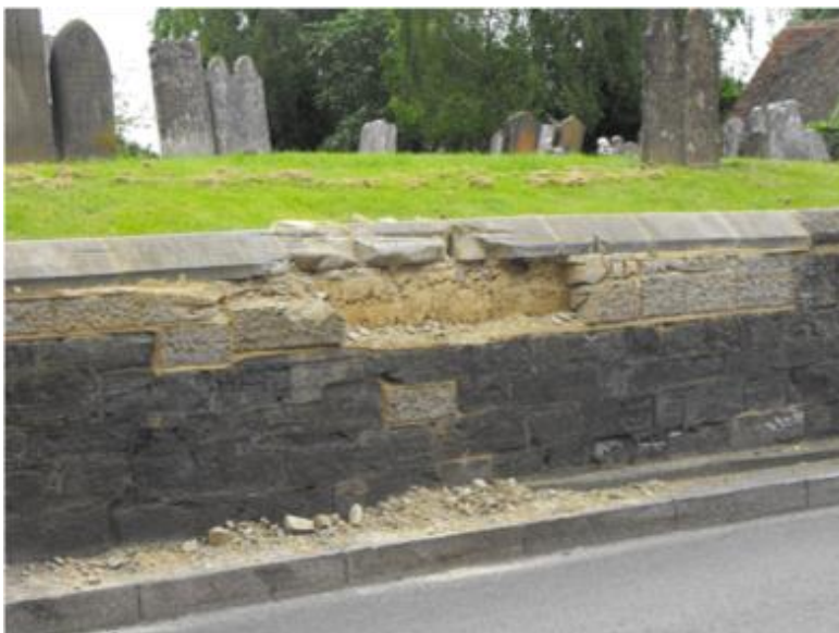
Figure 44 Damage to listed buildings
