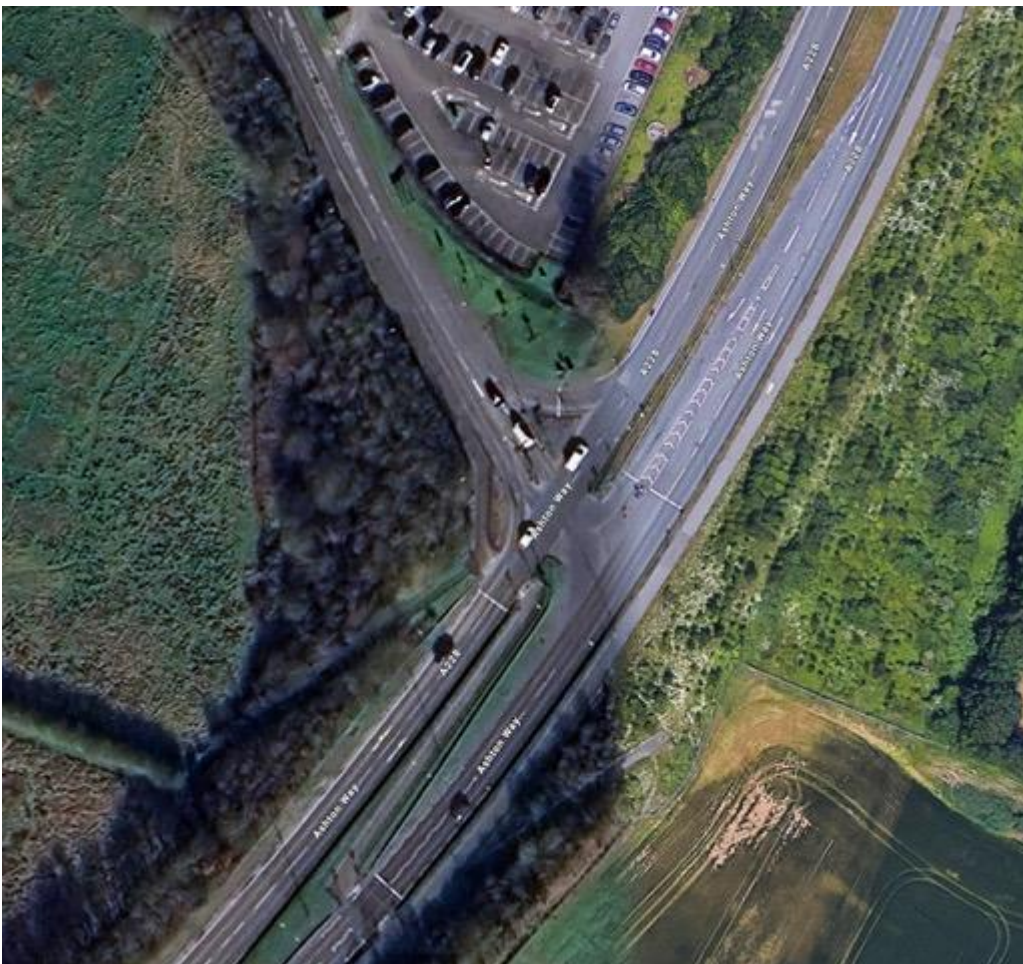
A228 Ashton way Traffic light controlled junction
