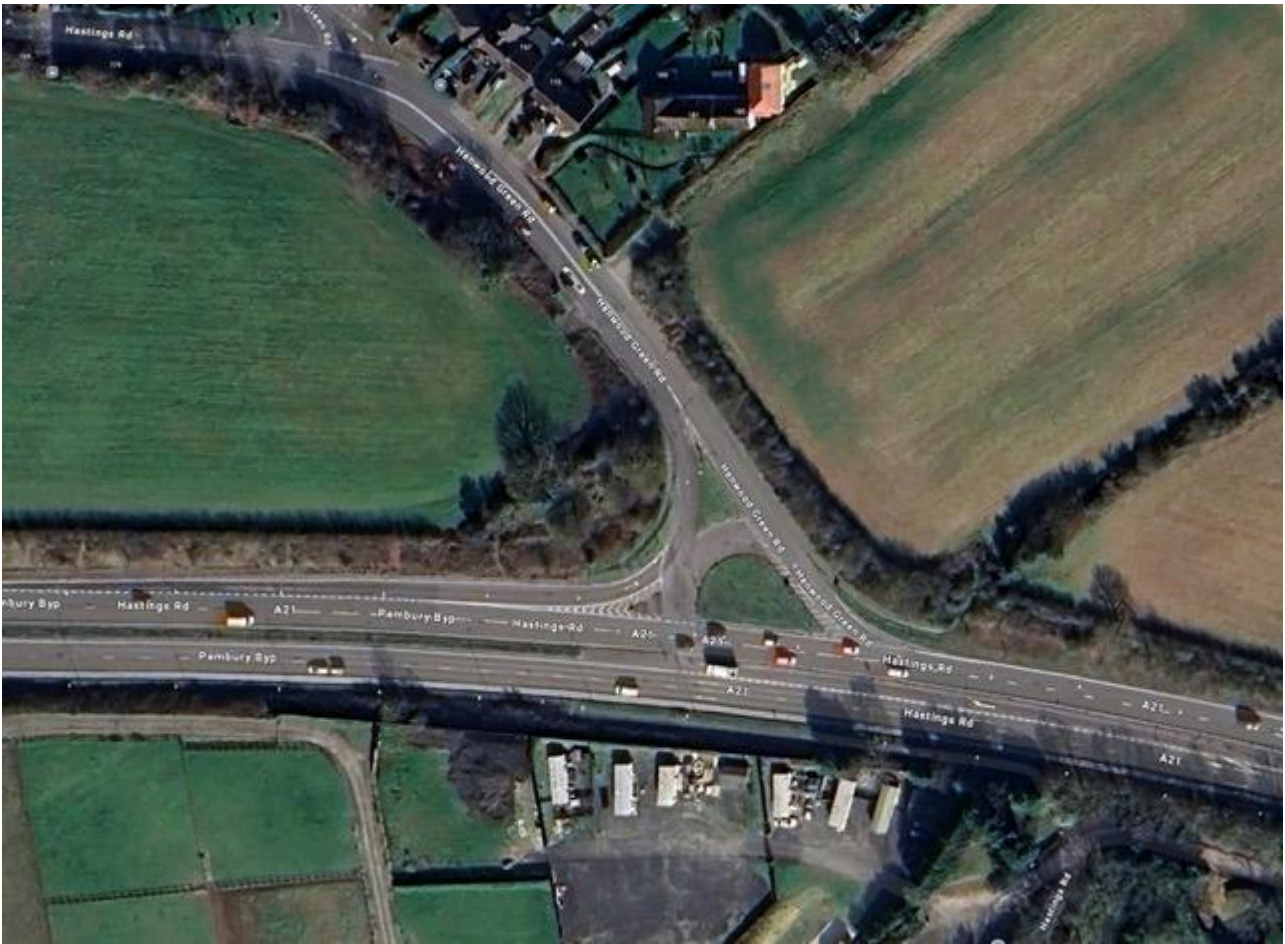
Existing Pembury South A21 junction
