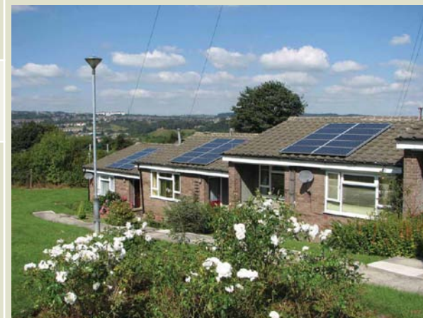
PV panels in Kirklees
