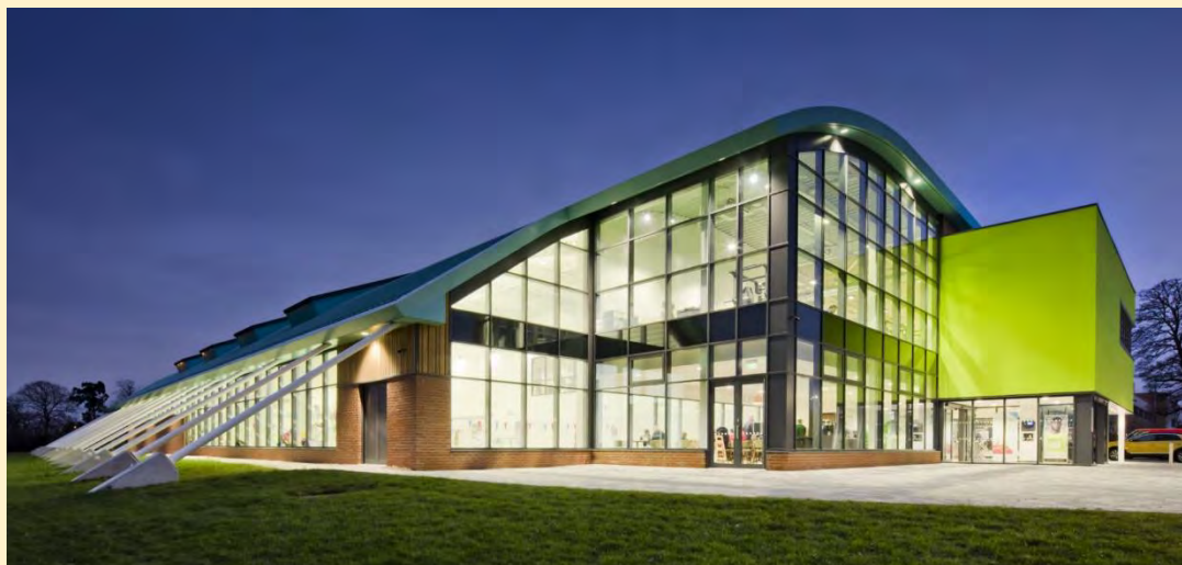
Figure 24: Morden Leisure Centre (Photo © GT3 Architects)
