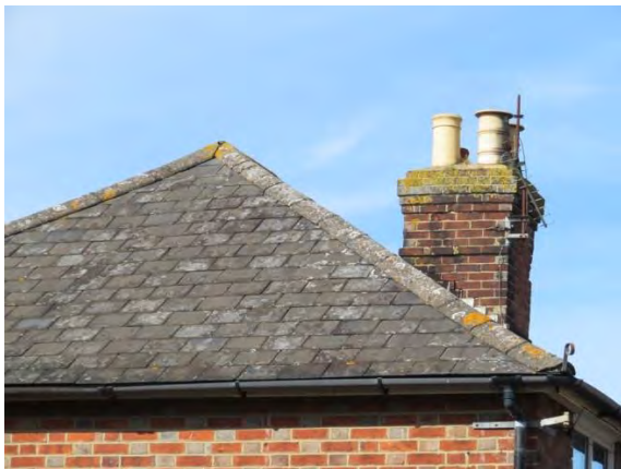
Roof tiles evident in central Paddock Wood
