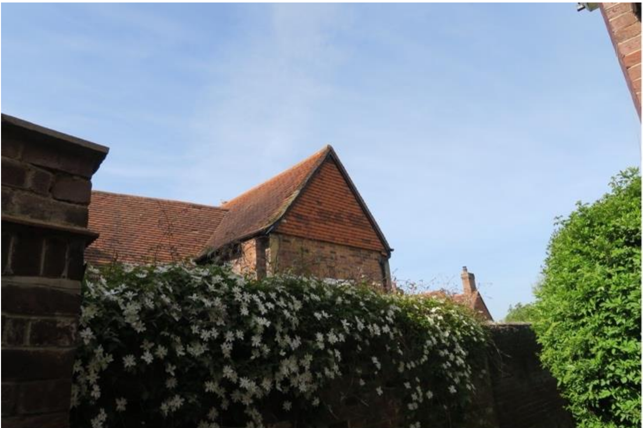
Figure 22: House showing typical tiled gable
