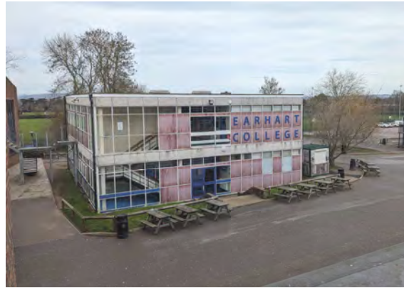
View of B Block
