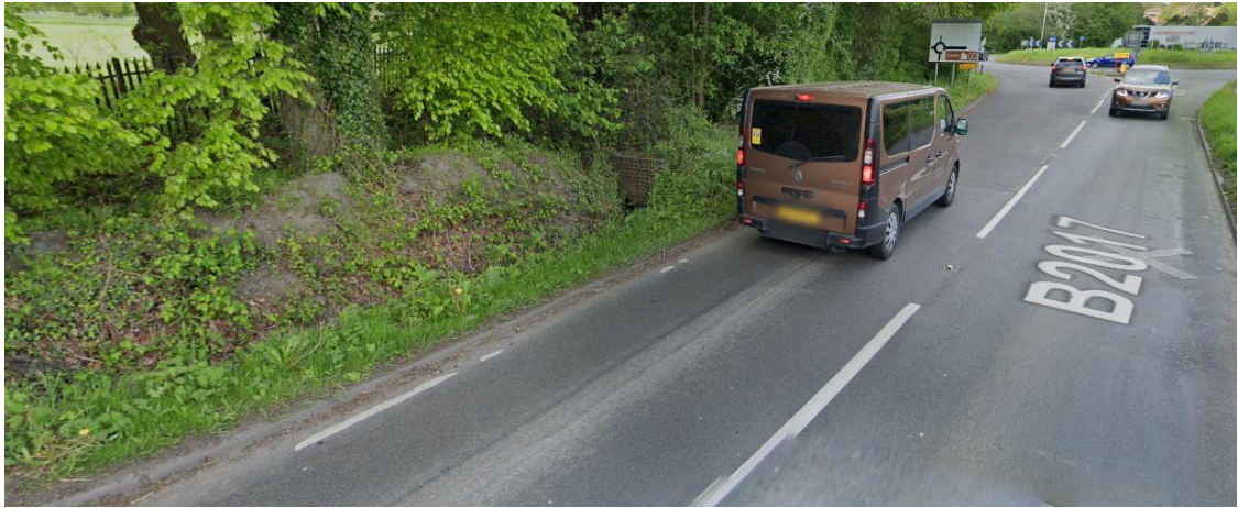
Existing drainage Infrastructure
